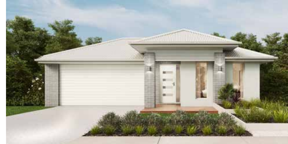
St Kilda Facade
