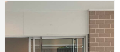
Fibre Cement Infill
